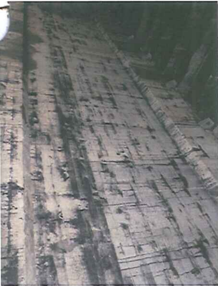
Figure 1-20: Girder 3 upstream face.
