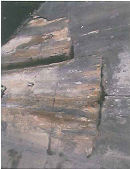
Figure 1-25: Left end abutment upstream wingwall.
