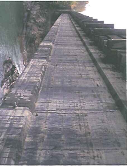
Figure 1-21: Girder 4 downstream face.
