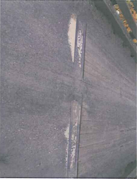
Figure 1-9: Right end approach joint.
