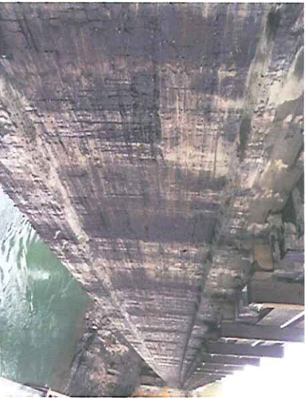
Figure 1-17: Girder 1 upstream face.
