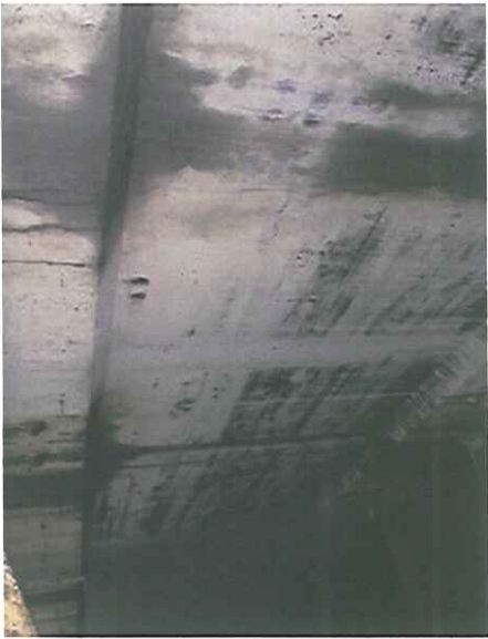
Figure 1-19: Girder 2 downstream face.
